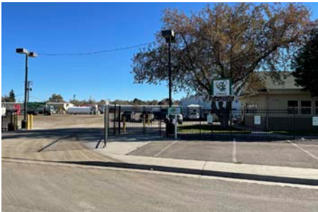
19 A concrete pumping business is located at South Windermere and Radcliff Avenue.
