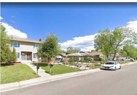
⑩ A variety of modest housing types are available in adjacent residential areas.
