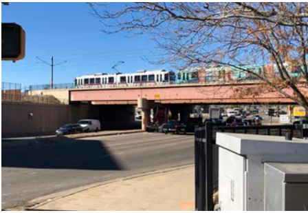
13 Oxford Avenue is difficult to cross as a pedestrian and feels unsafe. A new pedestrian bridge is being designed.
