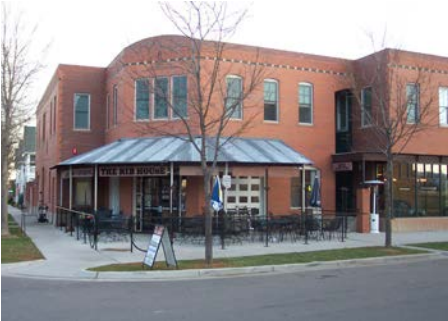
Adding neighborhood-oriented commercial uses, like restaurants, would help activate the southern area.
