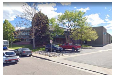
⑫ The Recreation Center is a great neighborhood amenity and destination.
