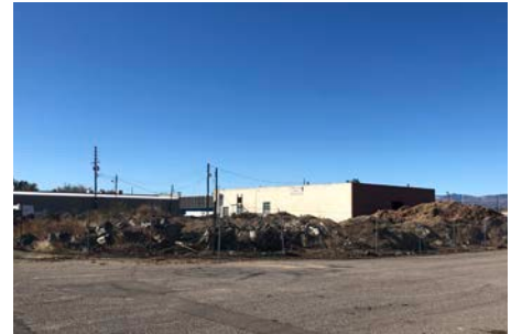
18 Some lots are used for storage or waste and appear to be abandoned and/or blighted.
