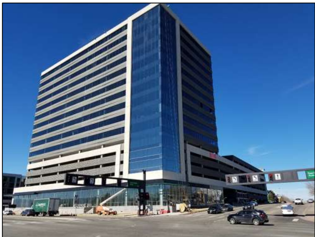
Belview Station 15 Stories, ~190 Feet
